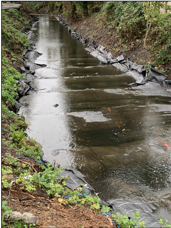
Figure 3. Reactive mat in the Lieve after construction
